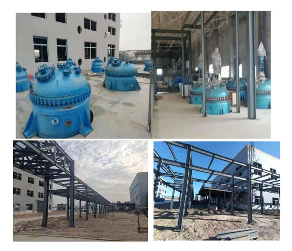
Photographs of the main base reactors and pipeline bridges are shown above.
