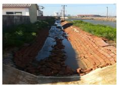
Flooding Damage to Aqueduct
