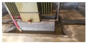
Flooding Damage to Equipment
