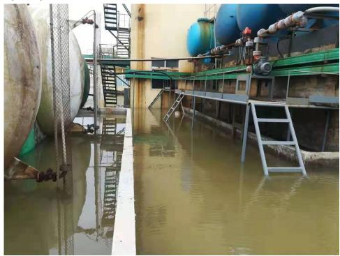
As can be seen from the photos above titled Lakima #3 and #4, the flooding damaged our factoryNo.7. However, since most of the equipment was raised, the damages were relatively easy to repair.
